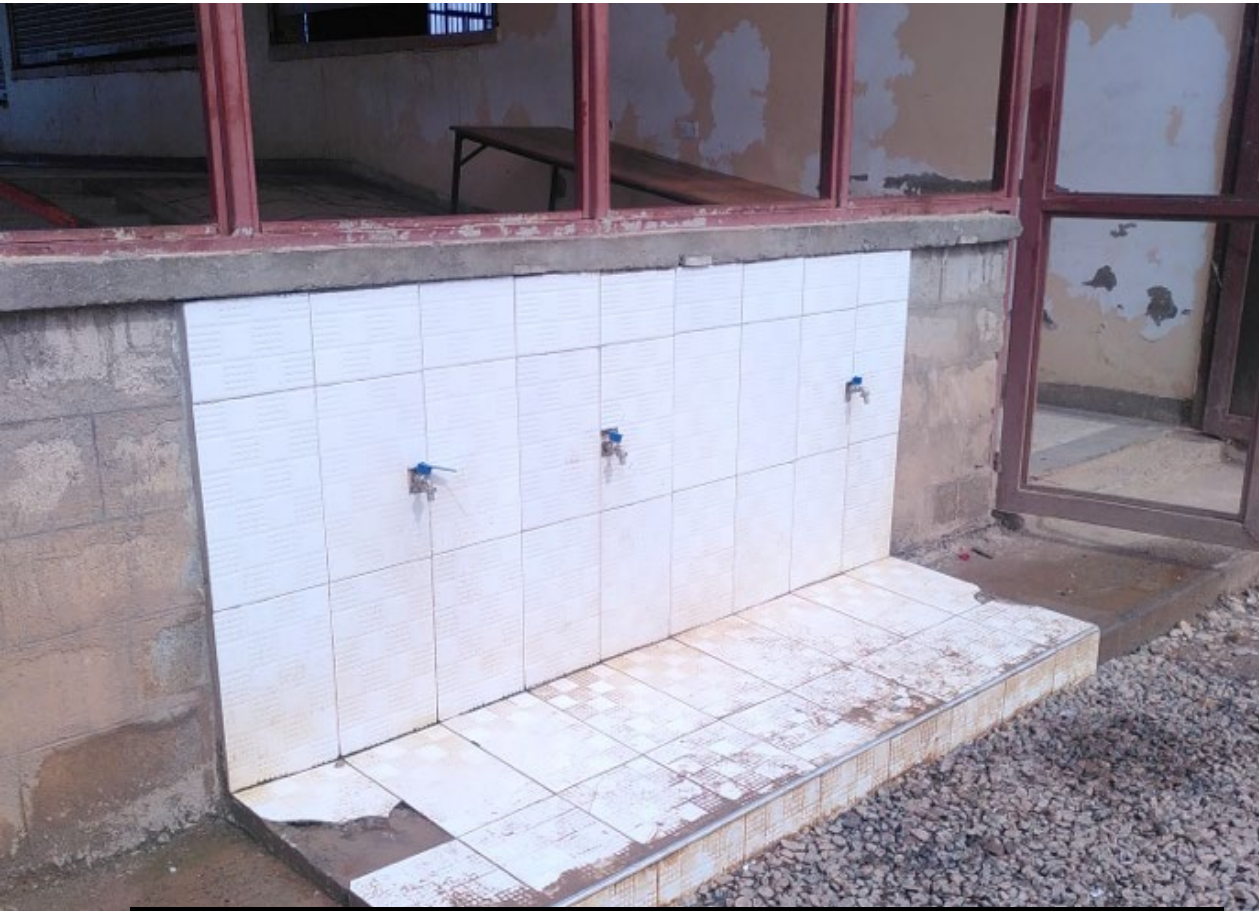
Public Stand Pipes (PSPs) with taps Source: Sandec
